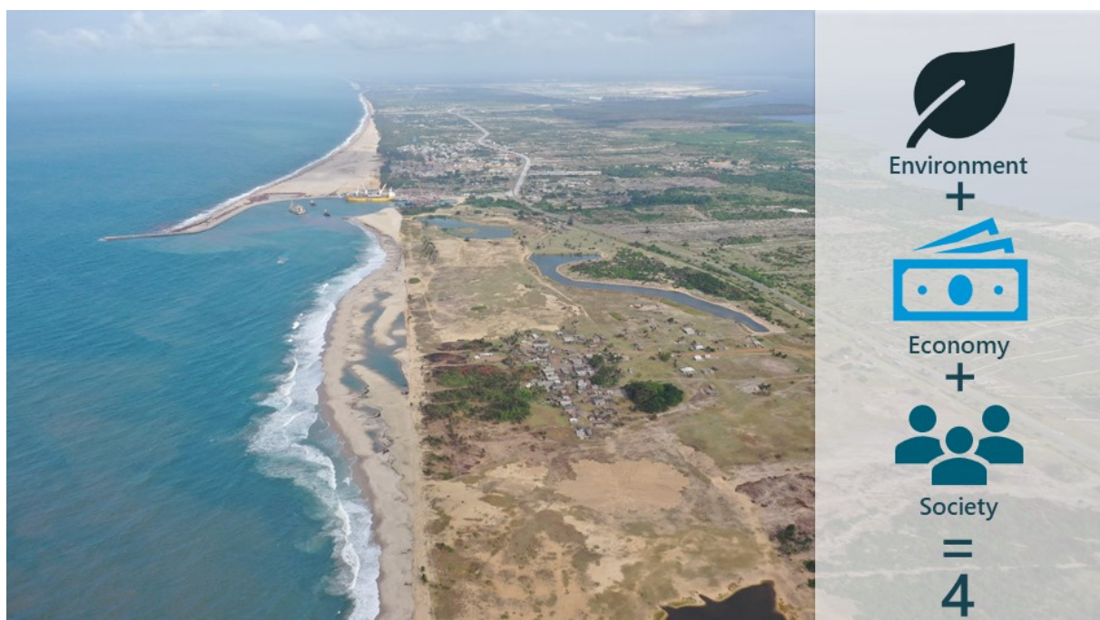
Figure 1 Systems Approach for Port Development - Sandbar Breakwater (Lekki, Nigeria)
