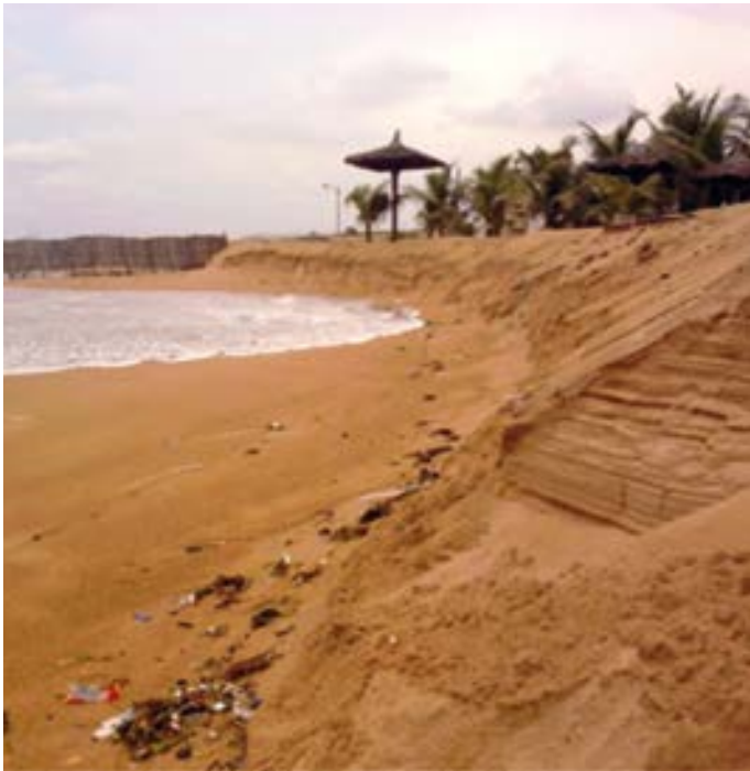
Important erosion (reflexive beach) in front of the port (Source, MOLOA's country office in Benin)
