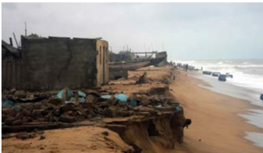
Strong erosion on the lido of Grand Popo (source MOLOA country branch of Benin)
