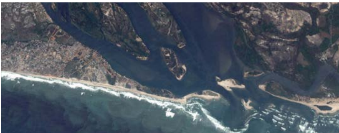
Ada shoreline protection project-Right bank of Volta mouthpiece, building of 7 groynes finalised in 2013 (Google Earth 2015)
