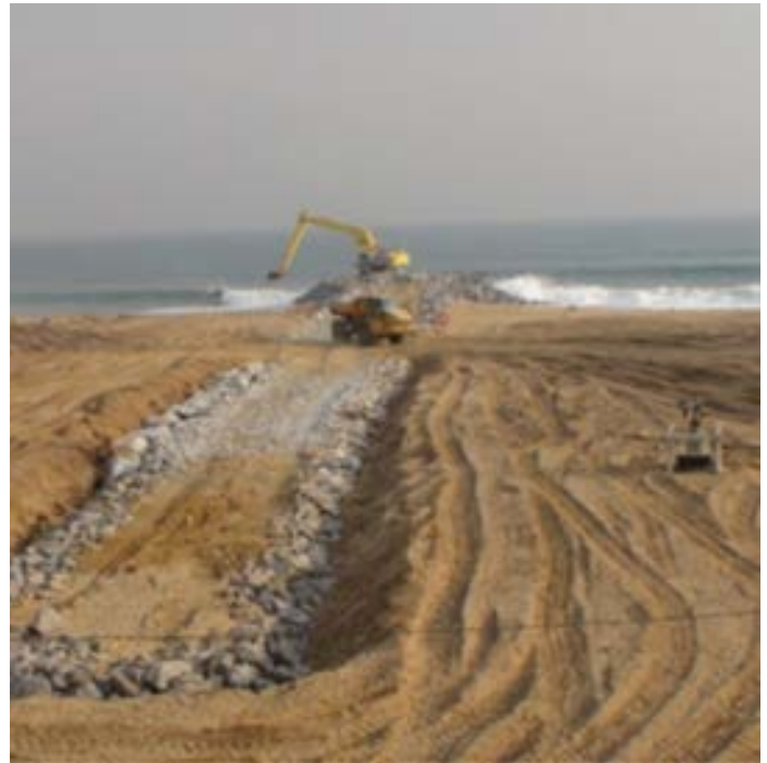
Development of the spurs system west of the port of Cotonou (source: MOLOA's country office in Benin)
