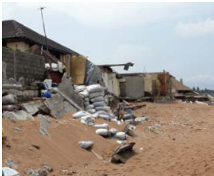
Destruction of upper-beach installations East of these installations of the mouth of the port's channel access (MOLOA)
