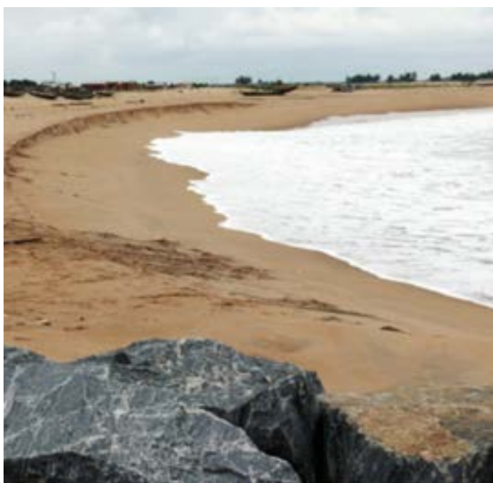
Resumption of erosion between the groyne of Keta planning (Formation of a berm at the top of the beach)
