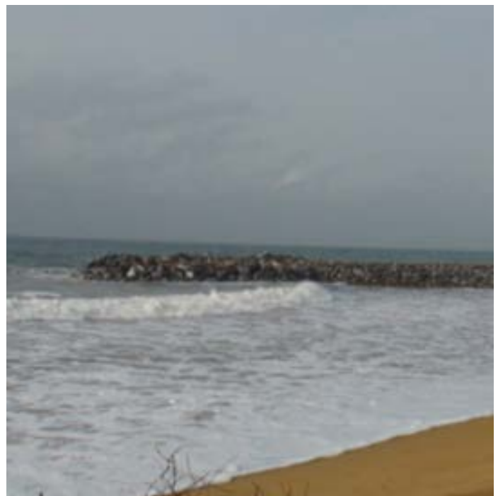
Development of the spurs system west of the port of Cotonou (source: MOLOA's country office in Benin)
