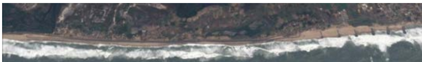
Protection works building of the coastal road between Salo and Angola (2010-2013) on the left bank of the Volta
