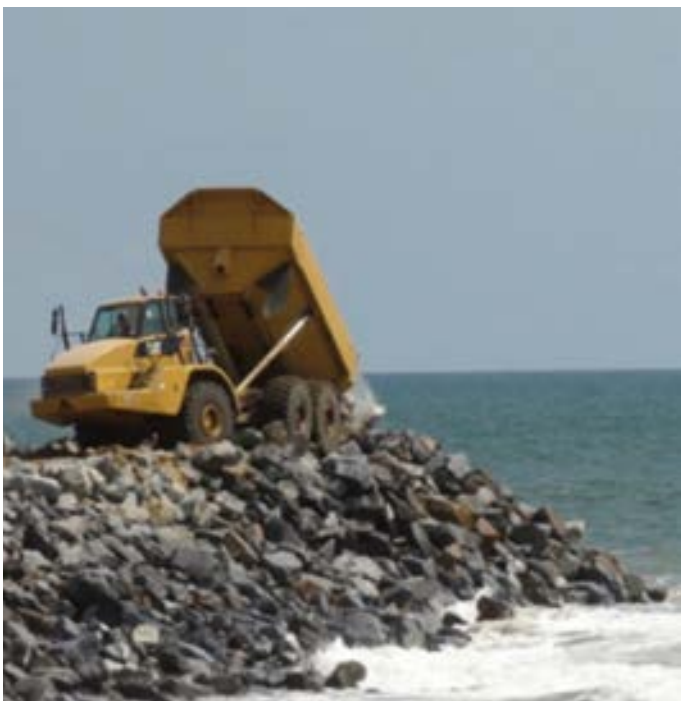
Development of the spurs system west of the port of Cotonou (source: MOLOA's country office in Benin)
