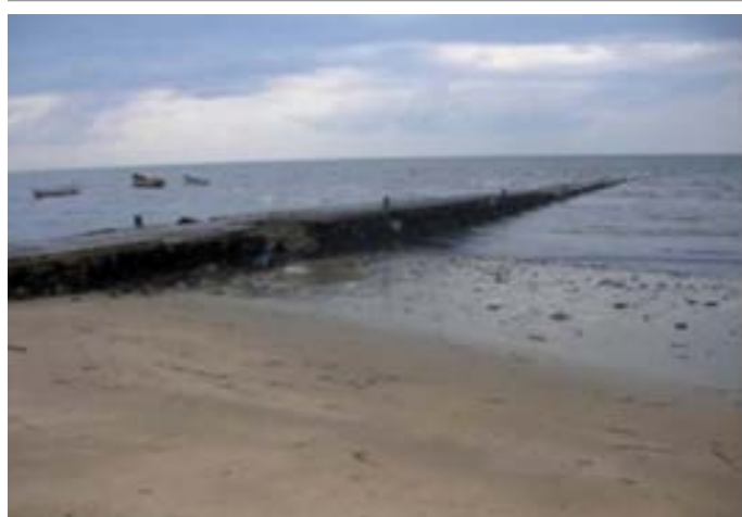
On the left, former Shenge jetty destroyed by erosion, On the right, new infrastructure (source: SDLAO case study).
