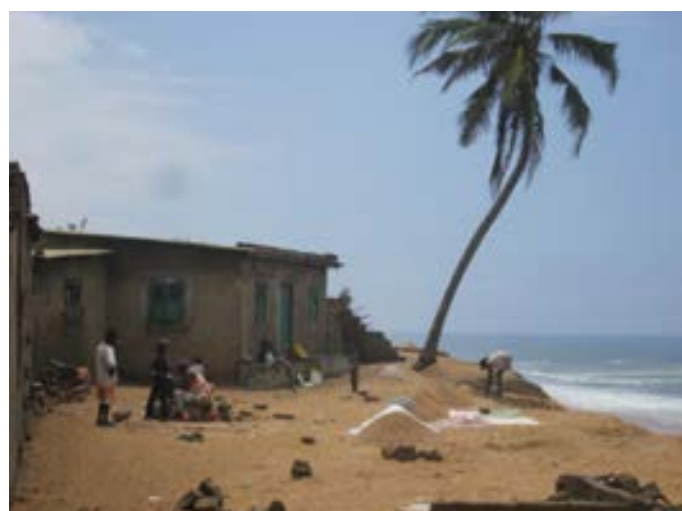
Coastal erosion in the east of the port of Lomé
