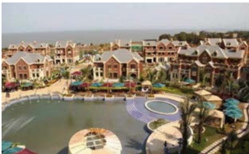
New housing (Diamond Piazza), in the Kipé District, Conakry
