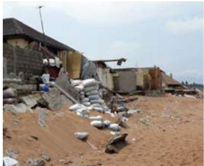
Destruction of upper-beach installations East of these installations of the mouth of the port's channel access (MOLOA)
