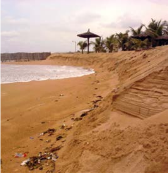
Important erosion (reflexive beach) in front of the port (Source, MOLOA's country office in Benin)
