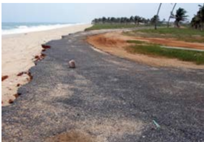
The effect of erosion in the Ada sector (Source: MOLOA Ghana country branch)
