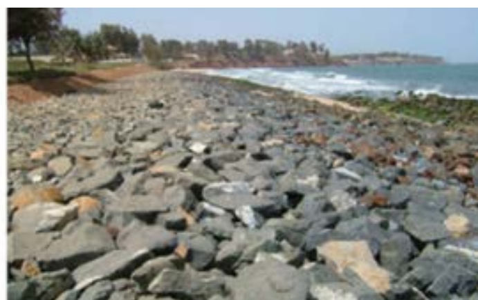
Armouring at Cape Point (source: SDLAO case study)
