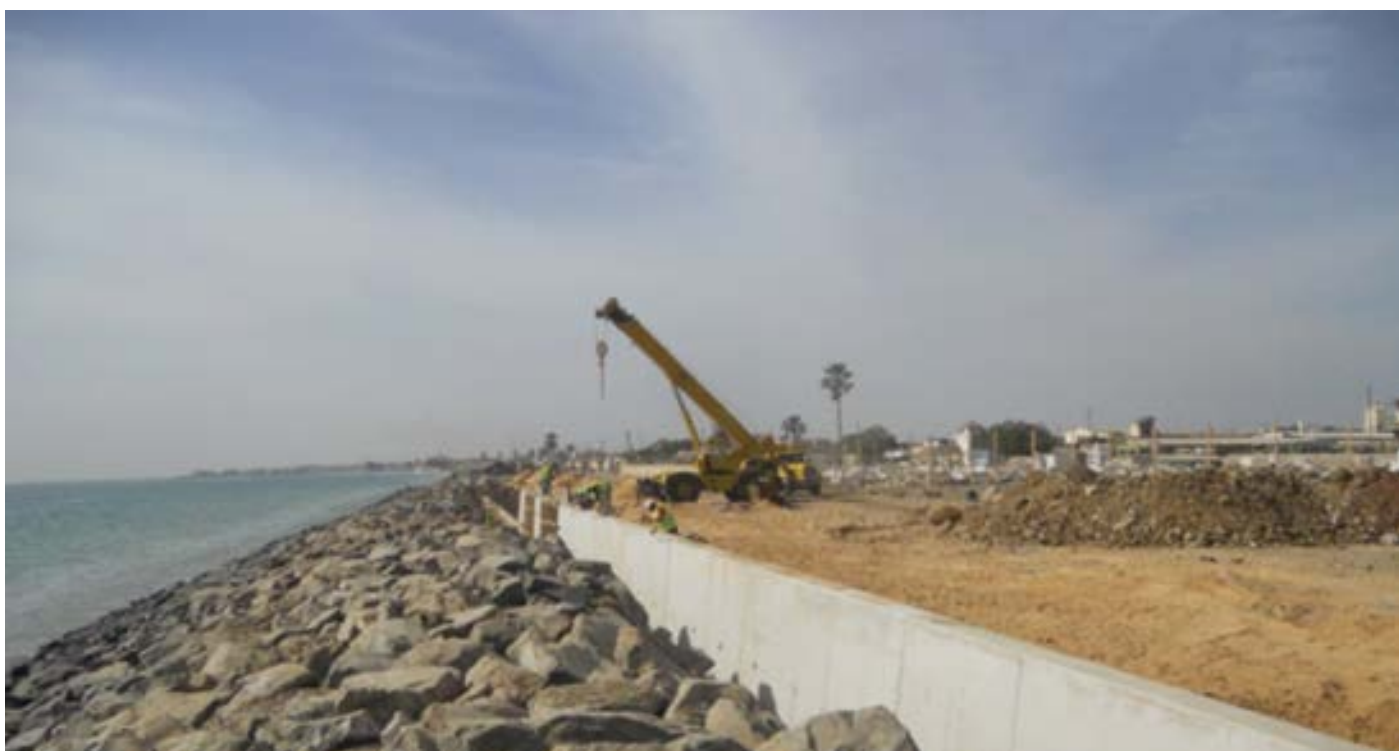
Building of Thiawlene dyke in 2012
