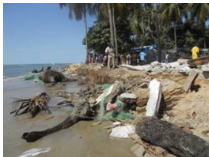
Erosion on Casamance islands (Karabane, March 2013) source MOLOA country branch in Senegal.
