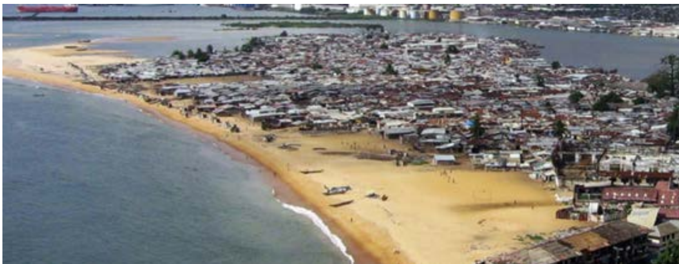
Precarious settlements of fishermen at West Point (source: SDLAO national diagnostics Liberia)
