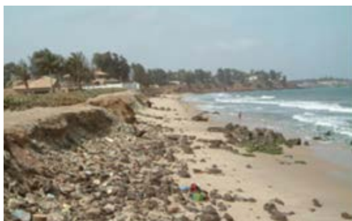
Armouring at Cape Point (source: SDLAO case study)
