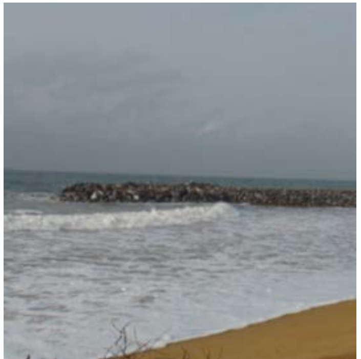
Development of the spurs system west of the port of Cotonou (source: MOLOA's country office in Benin)
