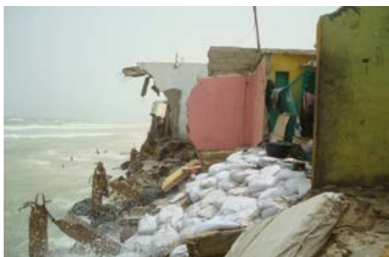
Collapsed houses in Guet Ndar following wave assaults
