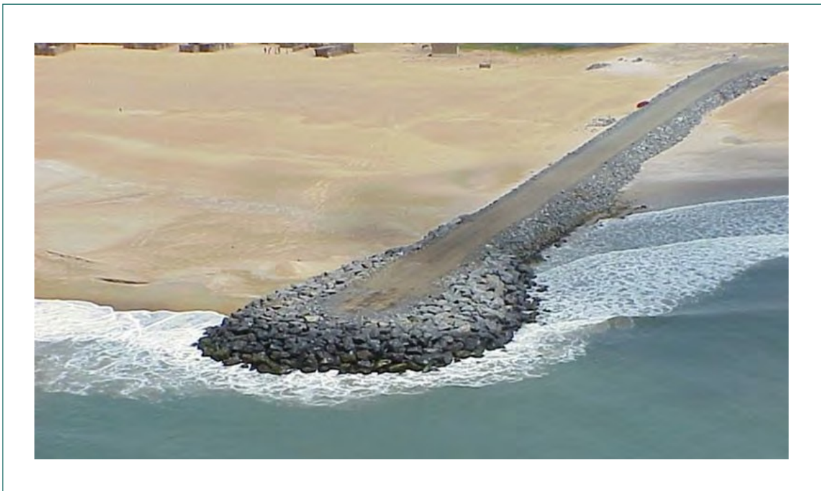
Figure 7. View of One of the Six Groynes Built Near Keta in Ghana for Longitudinal Crossing
