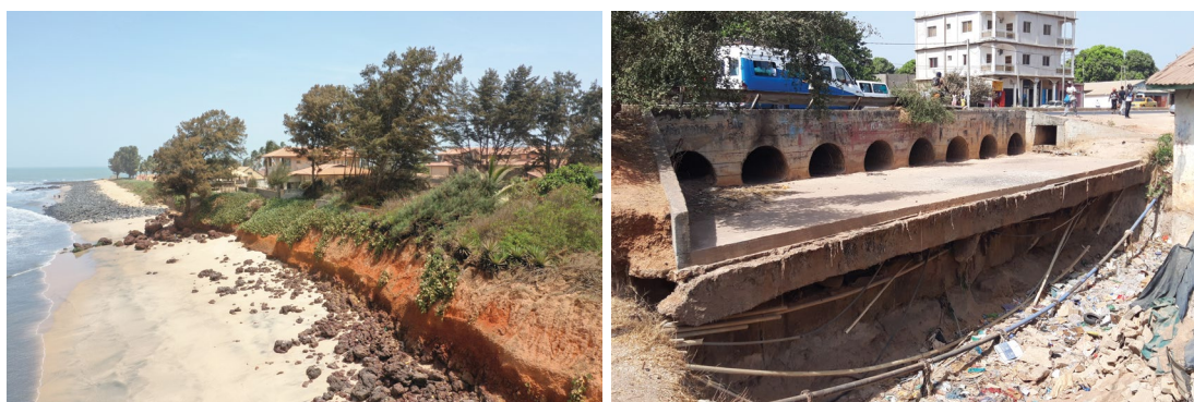
Figure 1.1 Erosion and coastal protection in Bakau (left) and a large culvert in Tabokotoh damaged by urban flooding (right)
