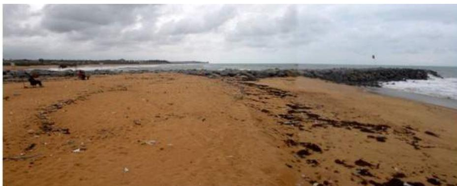
**Figure 4.9** Creek created by erosion phenomena downstream the groyne field (photo Laïbi, 2015).
