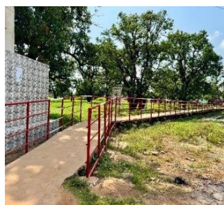
5 — Sukuta Nema, The Gambia — Ramps and footbridges on the Kotu stream: zero flooding in 2025.
