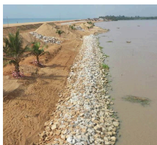
6 — Gbèkon, Benin — The bank of the Mono River, stabilized then revegetated.
