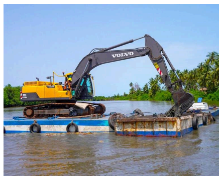
3 — Gbaga channel, Togo-Benin — Water flows again in the channel dredged by both countries.
