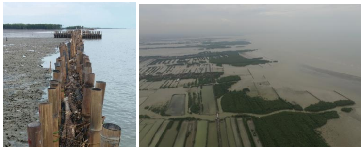
Figure IV.11 Left: Permeable structure a few months after construction with sedimentation at the landward side (to the left). Figure right: drone photo of the project area with at the left are the aquaculture ponds and in the middle the remaining mangroves. The straight lines are the permeable structures with sedimentation landward
