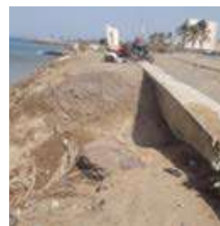
The erosion of coastal road formations is largely dependent on storm water management (Source: MOLOA country branch of Senegal)
