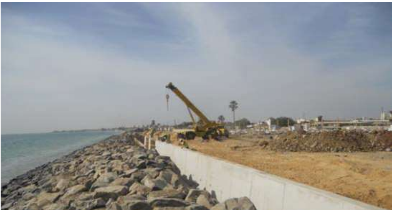
Building of Thiawlene dyke in 2012
