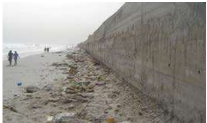
Protecting wall construction in progress in Mbao (Source: national Diagnostics)
