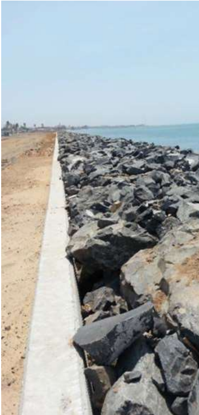
Dyke of Thiawlene (cost > 3 000 000 000 CFA)
