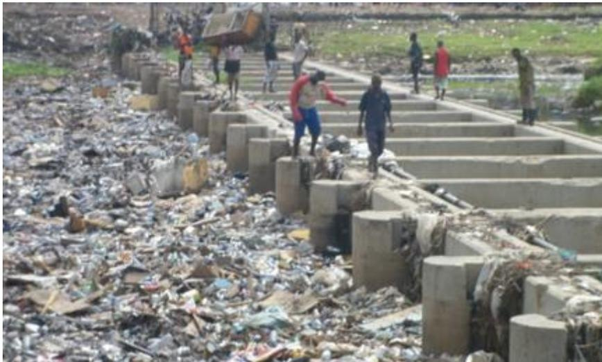
Figure 9: Floating plastic waste overtopping the Lagoon interceptor weir
