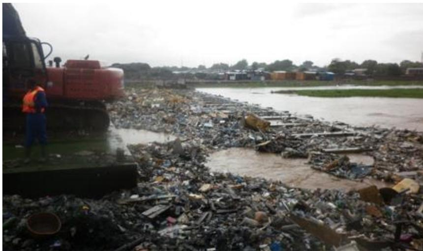
Figure 10: Dredging of plastic waste from the Lagoon interceptor weir
