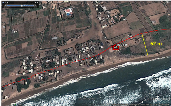
PHOTO 2 The shoreline of Baguida receded by 62 meters between 2011 and 2015
