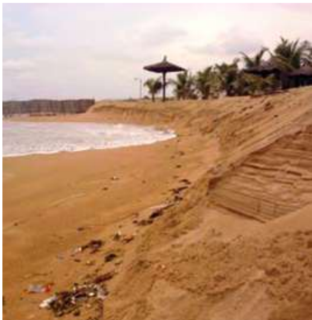
Important erosion (reflexive beach) in front of the port (Source, MOLOA's country office in Benin)
