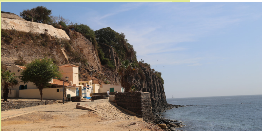
Cliff stabilisation in Gorée Island, Senegal. Photo: Madjiguene Seck/ World Bank
