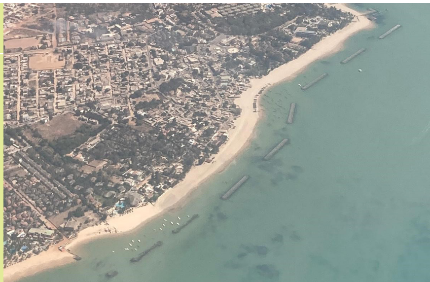
Breakwaters in Saly, Senegal. Photo: Senegal World Bank funded Tourism Project (PDTE)
