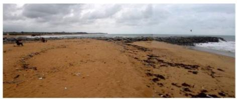
Figure 4.9 Creek created by erosion phenomena downstream the groyne field (photo Laïbi, 2015).
