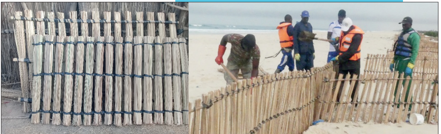
Photo 1 : Installation des typhavelles Photo 1: Installation of typhavelles
