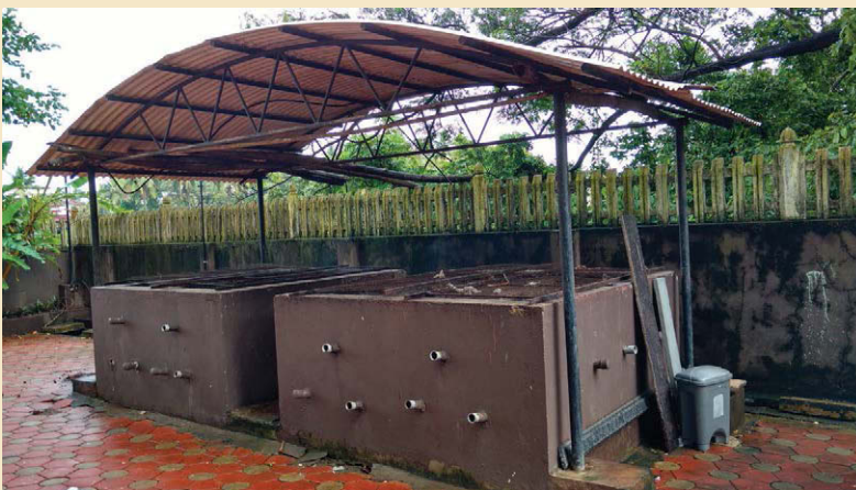
Photo 7.8c Decentralized Composting Units in Panaji, India
